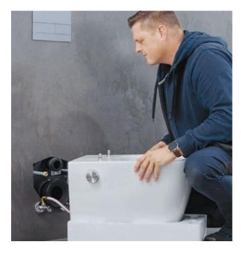
On the wall in a flash: TECEneo is delivered in installation-friendly packaging. For the water connection, TECEneo is pushed against the wall without straining your back, then lifted against the wall and firmly fixed using concealed clamping wedges.
